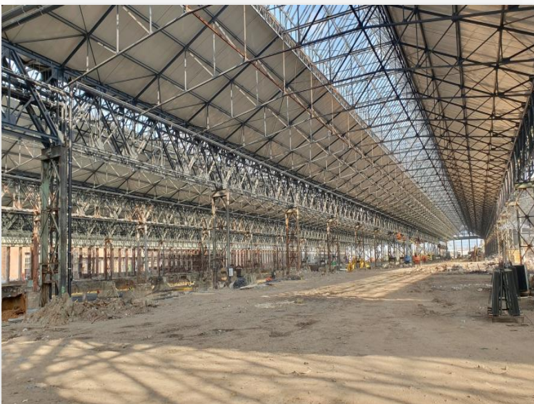
Hala Laminor (2019) – Interior
